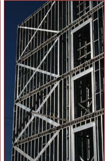
Fig. 3: Shear walls should be stacked vertically.
