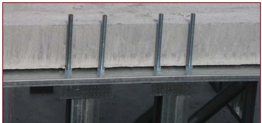
Fig. 2: Sheathing should not be attached directly to the StiffWall Column. Attach the sheathing to the adjacent studs.
