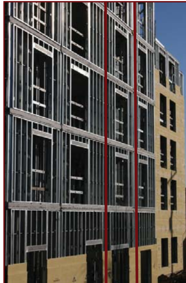
Example of framing aligned vertically. The red lines trace the axial load vertically from the roof to the foundation.
