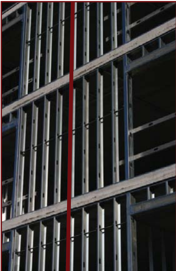
Example of framing aligned vertically. The red lines trace the axial load vertically from the roof to the foundation.
